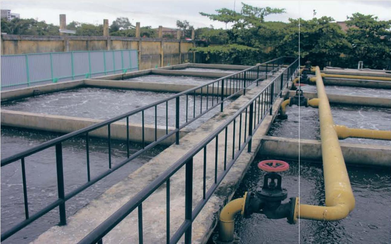
Figure 1: Activated sludge in the wastewater treatment plant of a textile company in Da Nang, Picture: Nguyen Minh Tan
